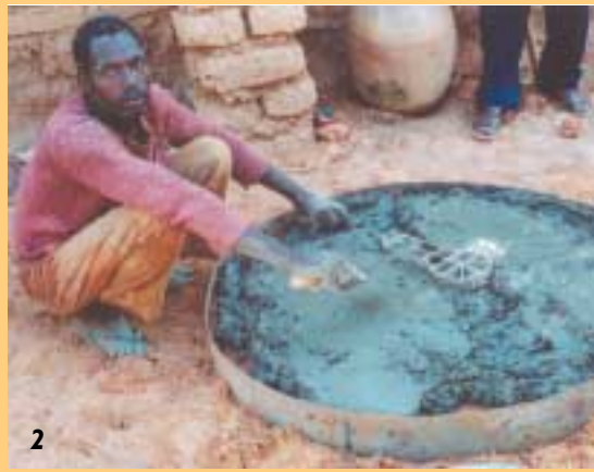
(1) A man makes a mold for a slab with an iron form and local sand base. (2) The man casts the slab with cement reinforced with iron bars. (3) The finished latrine has a lid. (4) This pit was dug to about 4 m and lined with mud blocks. (5) This pit was plastered with cement.
