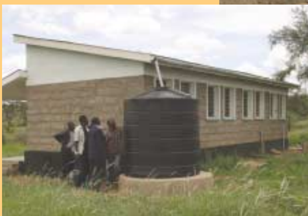
This tank at the clinic holds 3,000 L.
