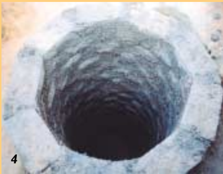
(1) A man makes a mold for a slab with an iron form and local sand base. (2) The man casts the slab with cement reinforced with iron bars. (3) The finished latrine has a lid. (4) This pit was dug to about 4 m and lined with mud blocks. (5) This pit was plastered with cement.
