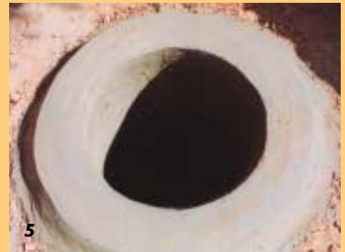
(1) A man makes a mold for a slab with an iron form and local sand base. (2) The man casts the slab with cement reinforced with iron bars. (3) The finished latrine has a lid. (4) This pit was dug to about 4 m and lined with mud blocks. (5) This pit was plastered with cement.
